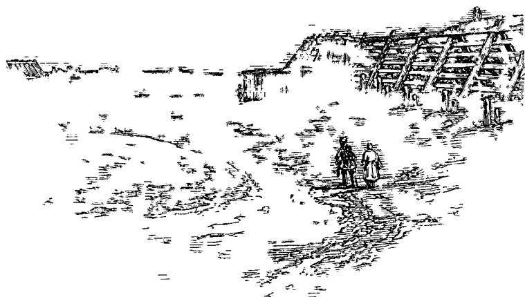
PUTRI WORKS, FROM THE NORTH.
