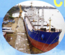
Jetty Service and Berthing Facility
