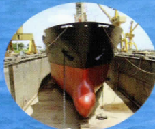
Ship Repair & Renovation
